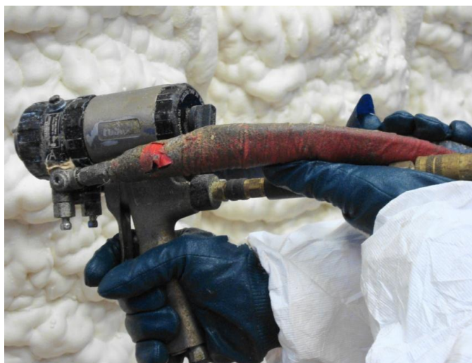
Figure 10: Fabric Gloves Coated with Nitrile
